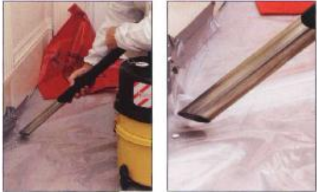
Vacuum clean carefully. It is easy to disturb asbestos fibres, make them airborne and breathe them in
