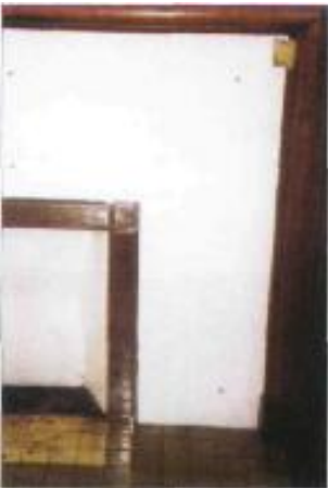
Asbestos insulating board (AIB) fire surround
