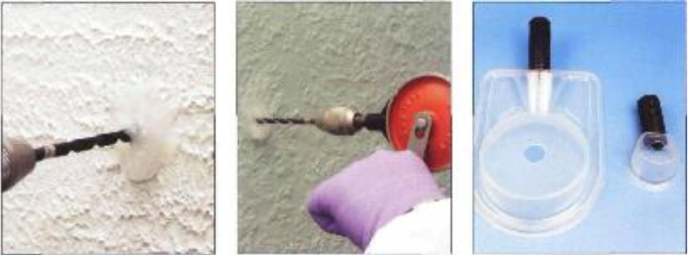
Drill through paste or foam or use a plastic cowl or other proprietary device with a Class H vacuum cleaner
