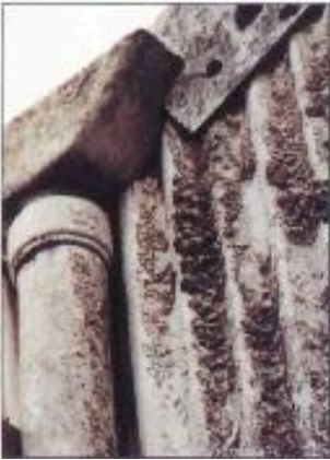
Moss and lichen growth on asbestos cement roofing and gutters
