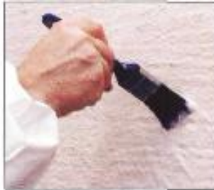
Sometimes it may be easier to wet the area using a brush or roller
