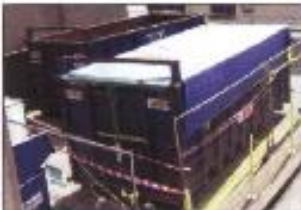
Use a lockable skip for asbestos cement sheets.
