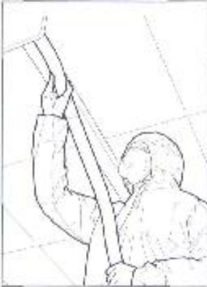
Cleaning inside the tube fitting with a Class H vacuum cleaner
