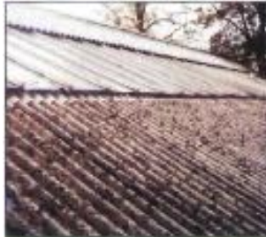
AC sheets used as roofing
