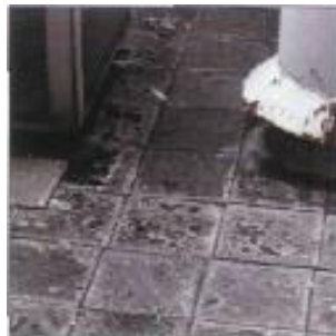
Asbestos cement tiles on a roof
