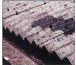
AC sheets used as roofing
