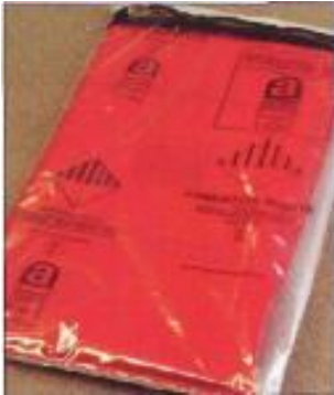
Double wrap the door in polythene sheeting with asbestos warning stickers
