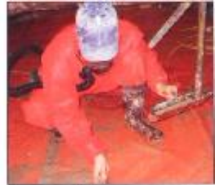
Over-wetting the material creates a waste slurry which will be difficult to clean up
