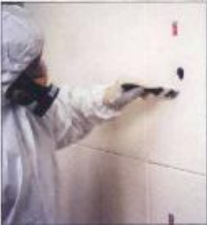
Seal the drilled edge with sealant
