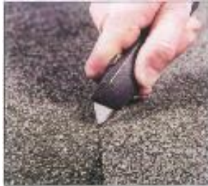
Cut and remove manageable sections
