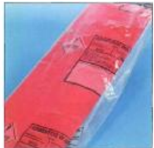
Cut the bolts while avoiding contact with the asbestos cement. Double-wrap large pieces in 1000-gauge polythene sheeting and seal with duct tape
