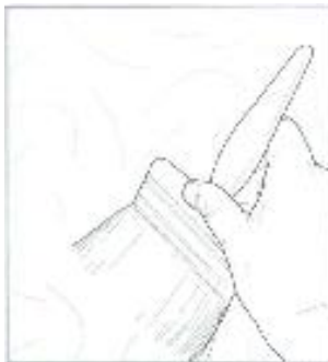
Gently brush on penetrating fluid, or dampen and loosen the coating with steam
