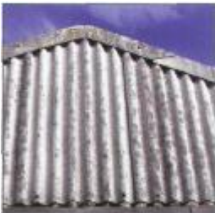
Cut the bolts while avoiding contact with the asbestos cement. Double-wrap large pieces in 1000-gauge polythene sheeting and seal with duct tape
