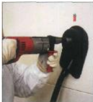
Control measures: Shadow vacuuming and using plastic enclosures as local extraction
