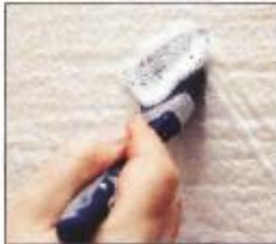
Paint sealant around the hole before you insert the screw. Use shadow vacuuming to control dust when removing screws
