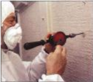
a26 tells you how to drill through textured coating
