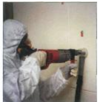
Control measures: Shadow vacuuming and using plastic enclosures as local extraction
