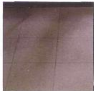
Interior floor tiles
