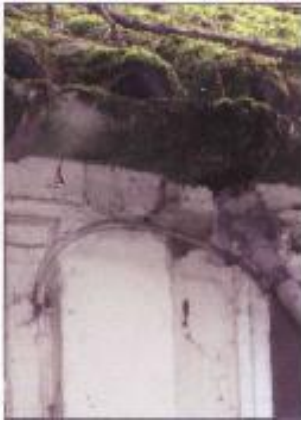
Moss and lichen growth on asbestos cement roofing and gutters
