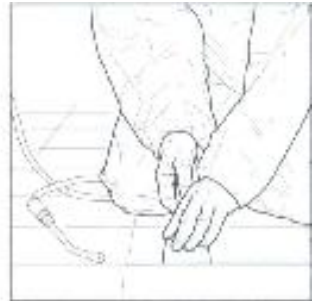
Spray water under the tiles to suppress dust as you lift them gently, avoiding breakage
