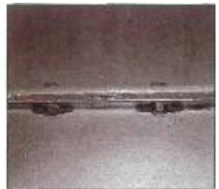
String gasket between metal sheets
